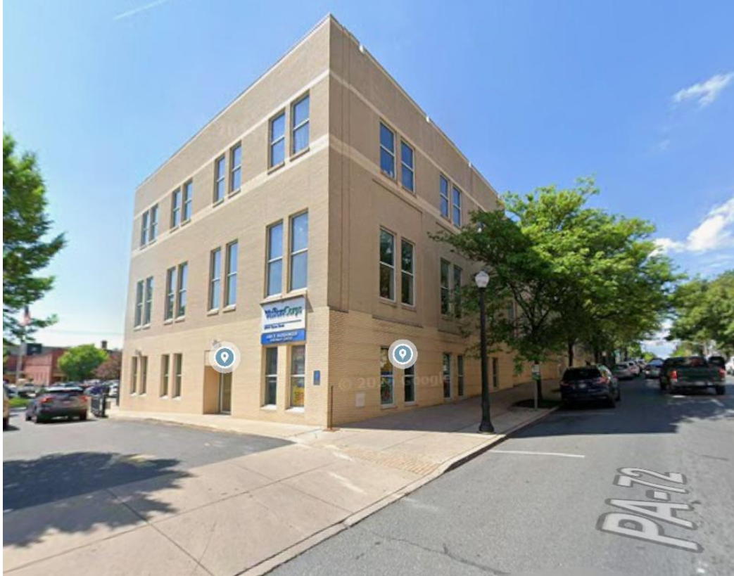
VisionCorps building located at 244 N. Queen St., Lancaster, PA.
